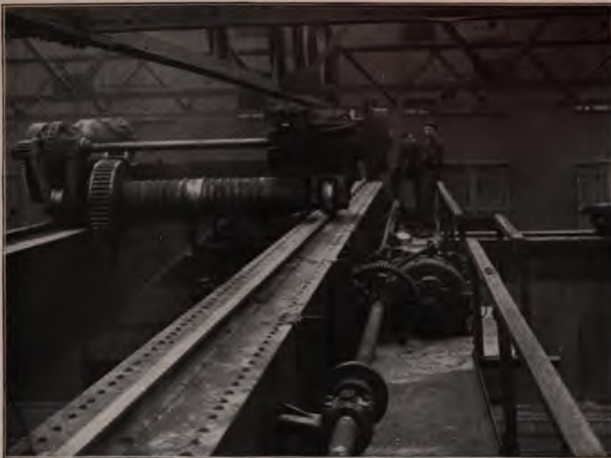
PLATE 7.—ELECTRIC TRAVELING CRANE BOUGHT ABOUT TEN YEARS AGO This shows open gearing, overhung gears, exposed couplings, etc.; the foot-walk on which the men are standing was placed on the crane after it had been installed
